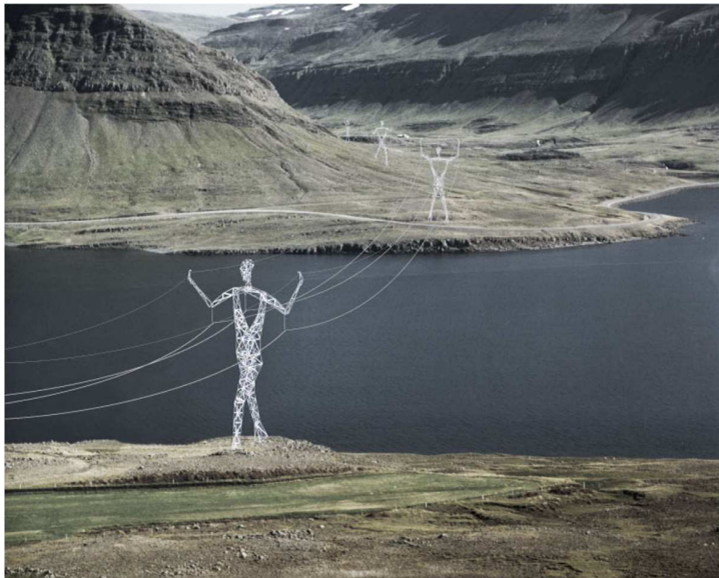
Figura 41 Land of Giants. Choi and Shine Architects, Islandia, 2008. Naturaleza interpretativa de la representación
